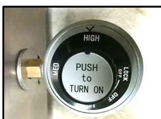
Fig. 3: Regulator Valve Lighting Position
